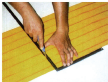
1. cut off the PVC strips
